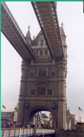
The Tower Bridge can be lifted up in order to let big ships through.
